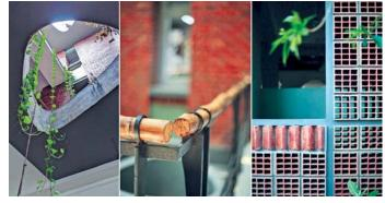
Natural and rustic features added into the detailing of railing and façade elements - light well, handrail detail, clay *jali* and perforations *Source: Vivek Venugopal*
